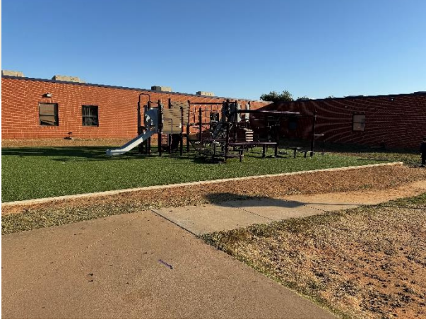
New playground structure at Grand Elementary
